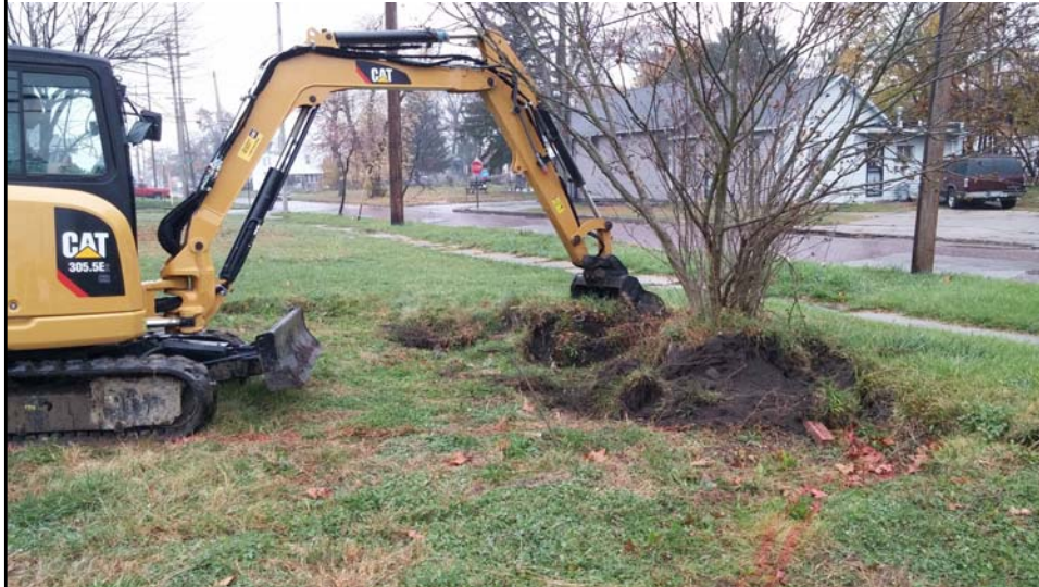
Rain garden construction – transplanting select existing vegetation
