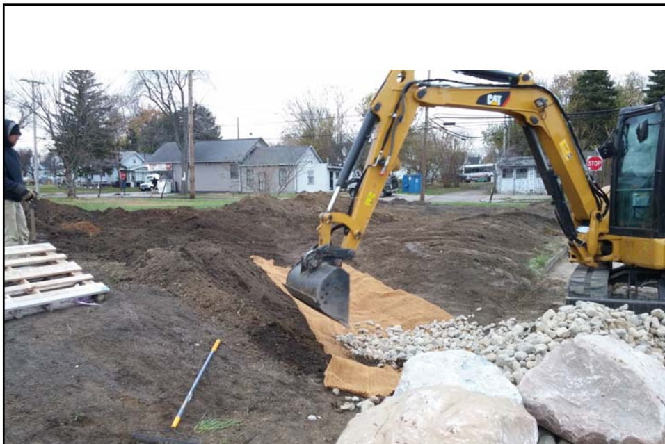
Rain garden construction – building rock channel inlet
