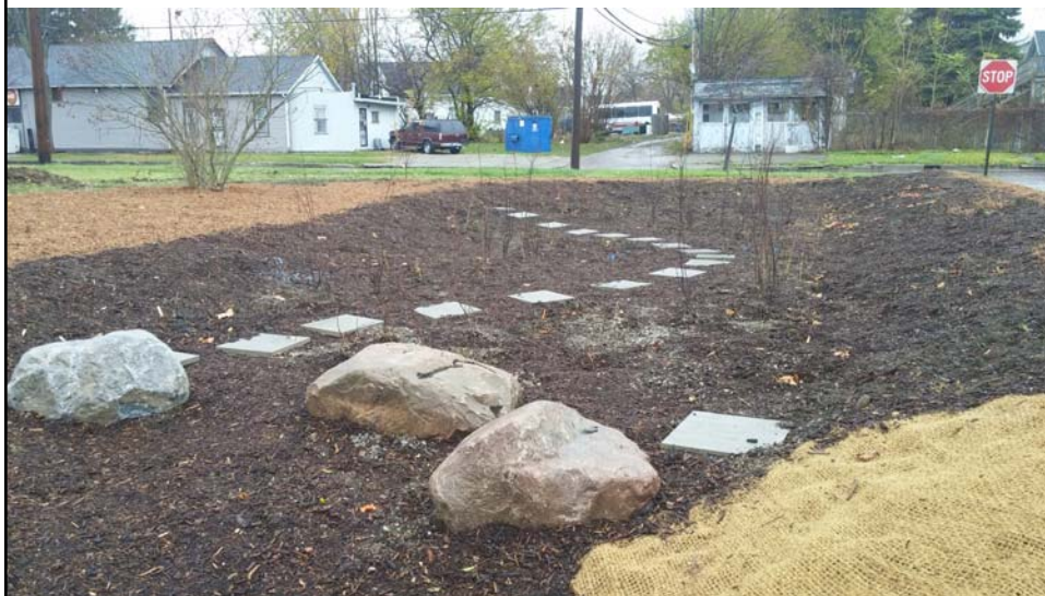
Finished rain garden complete with rocks, plantings, and stepping stones (November, 2015)
