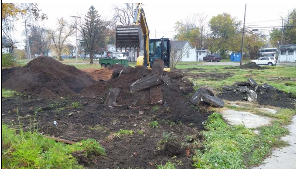
Rain garden construction – Existing parking pad was removed
