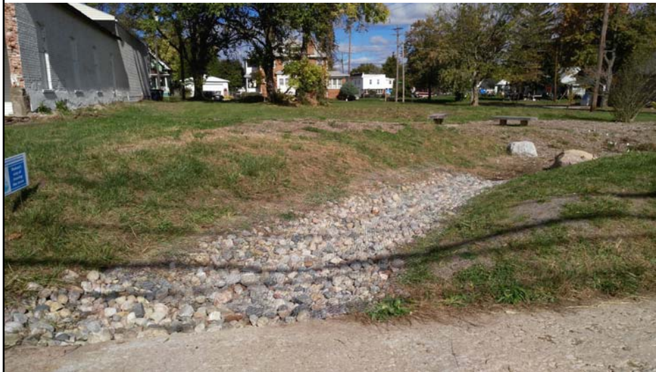
Rock channel stabilized with staked chicken wire to prevent vandalism
