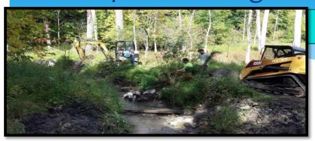
Improving erosion control in Hartman Ditch with mini-Bendway Weirs and plantings
