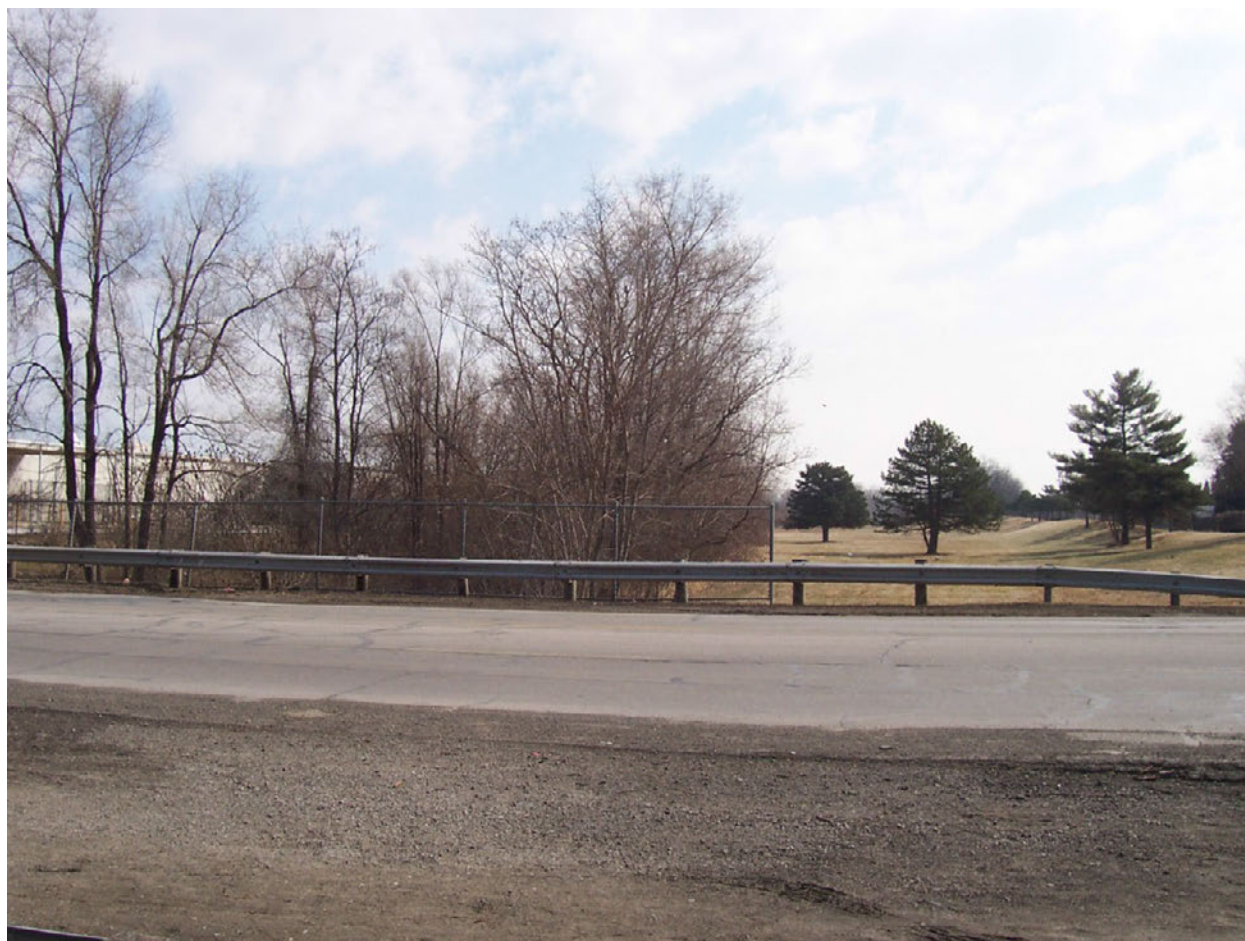
Figure 36. Lewis Avenue bridge over Silver Creek (facing east, downstream).
