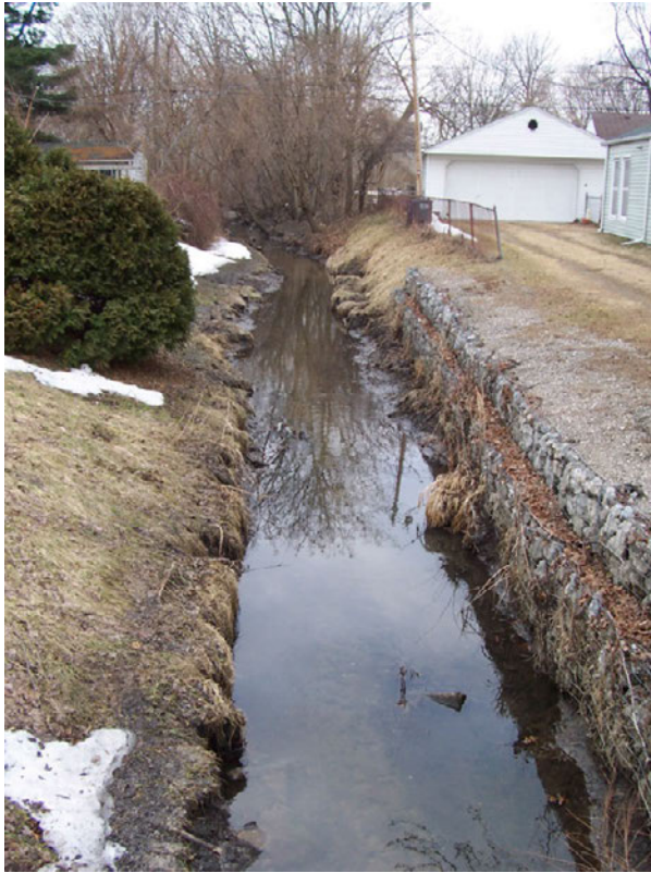
Figure 30. Ketcham Ditch at Adella Street (facing west, upstream).
