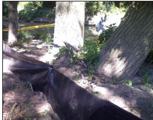
*Silt fences (black in foreground) were installed on land and silt curtains (yellow in background) in the water to control sediment leaving the construction site.*
