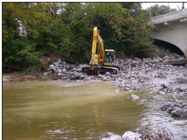
Heavy equipment was used to move the rock across the stream and to compact it.
