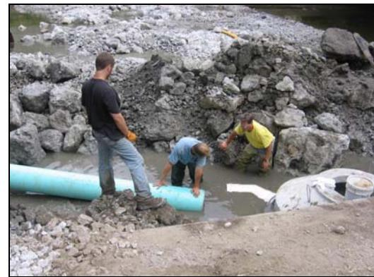
*New manhole and storm sewer pipe being connected to an existing storm sewer in the dam's west retaining wall.*
