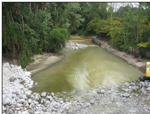
*Silt curtains were installed downstream of the second structure.*
