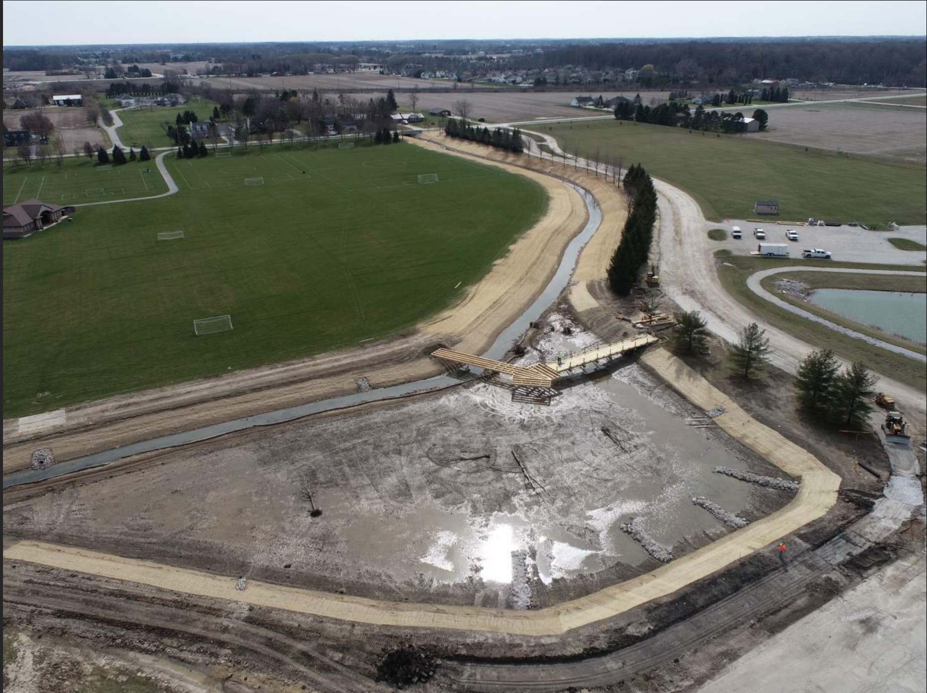
West Floodplain Area, Wolf Creek Stream and Floodplain Restoration Project, March 2024
