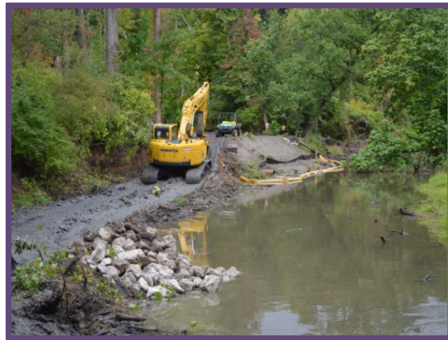
Construction begins by moving the stream bank material to position the LPSTP into a smoothed alignment.
