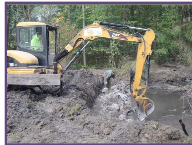
Excavator then positions the stone into the triangular shape, or otherwise if installing LFSTP. Behind the excavator’s work, Live Siltation is installed against the stone.
