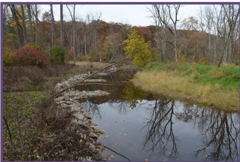
Image 3: LPSTP and Bendway Weirs at Camp Miakonda in Sylvania, OH. Kyle Spicer
