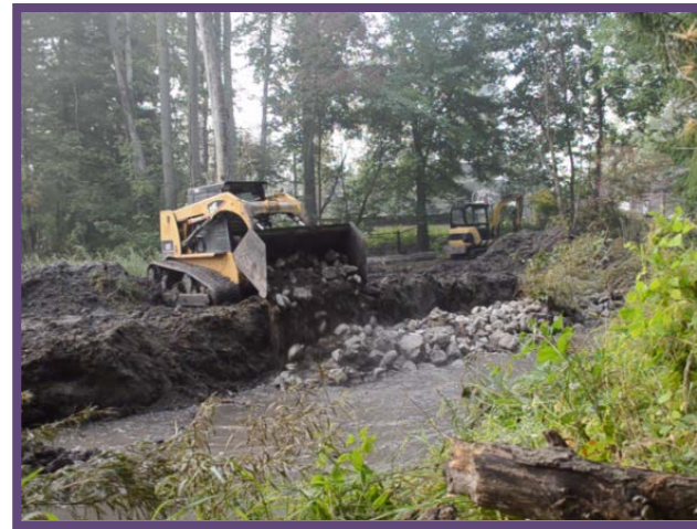
Stone is then deposited, depending on the size of the stream, over the bank with a skid loader or dump truck.
