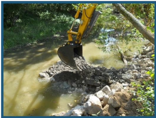
These BW in particular were heavily choked, to create a smoother surface for people to walk on and gain access to the river.
