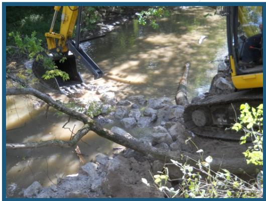
The BW is shaped as additional stone is placed on top. For medium – large streams, a majority of the stone is placed one bucket of well-graded stone at a time.
