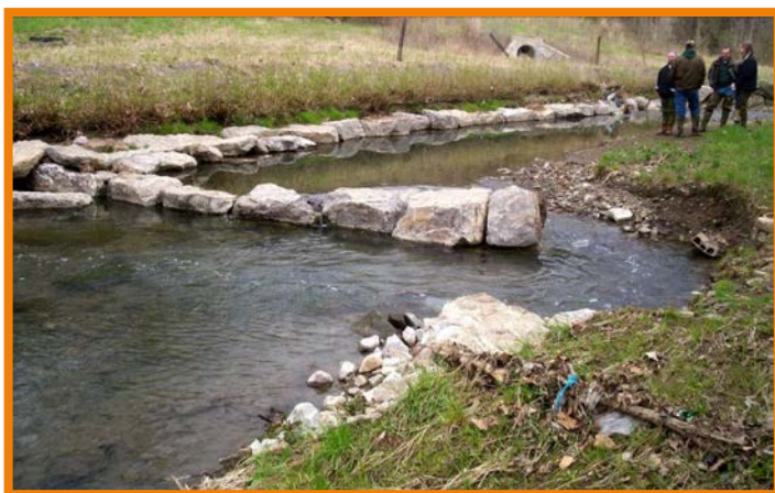
Image 1: A flanked grade control structure. Derrick
