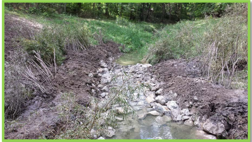
Image 2: Live Siltation installed along an Engineered Rock Riffle and Keys. Camp Miakonda, Sylvania, OH. Kyle Spicer
