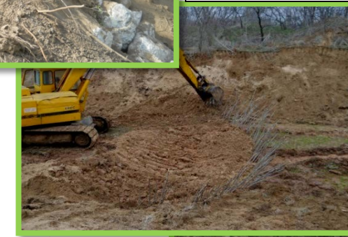
Vegetation is backfilled and secured; typically overfilled to accommodate settling soil. Now just add time!
