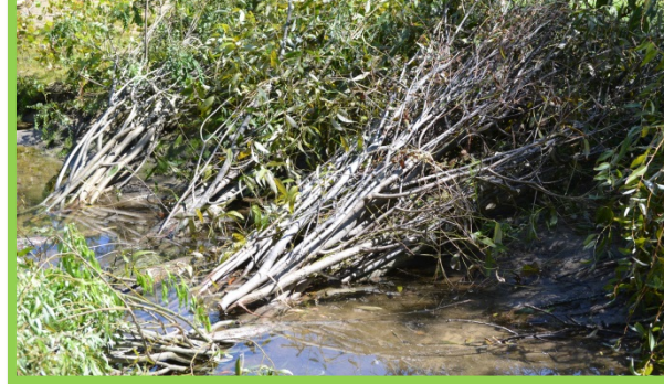
Plants are harvested, bundled, tied together, placed in the shade, and then soaked until installation.
