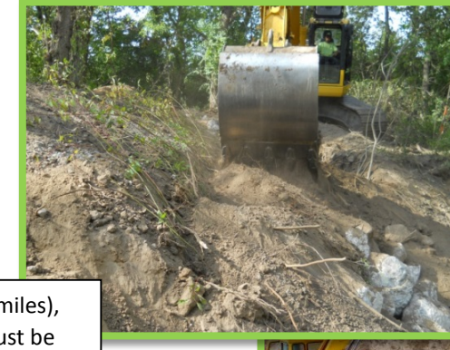
Vegetation is backfilled and secured; typically overfilled to accommodate settling soil. Now just add time!
