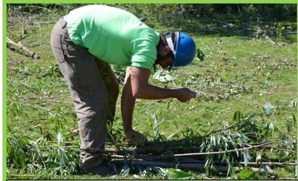
Plants are harvested, bundled, tied together, placed in the shade, and then soaked until installation.
