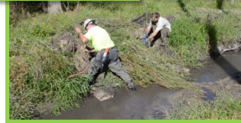
Plants are installed by hand after Keys are dug and before rock is installed.
