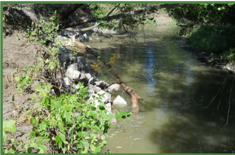
Image 3: Thalweg realignment Locked Log in Ottawa River at Camp Miakonda, Sylvania, OH. Kyle Spicer
