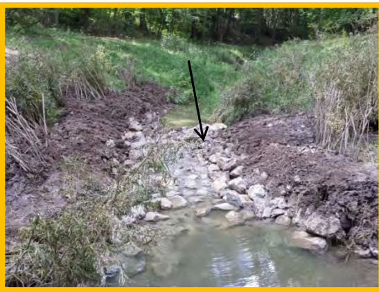
Image 1: ERR has a 20 to 1 slope on the downstream face for stability, to entrain air, for fish passage, and to dissipate energy. Camp Miakonda. Kyle Spicer.
