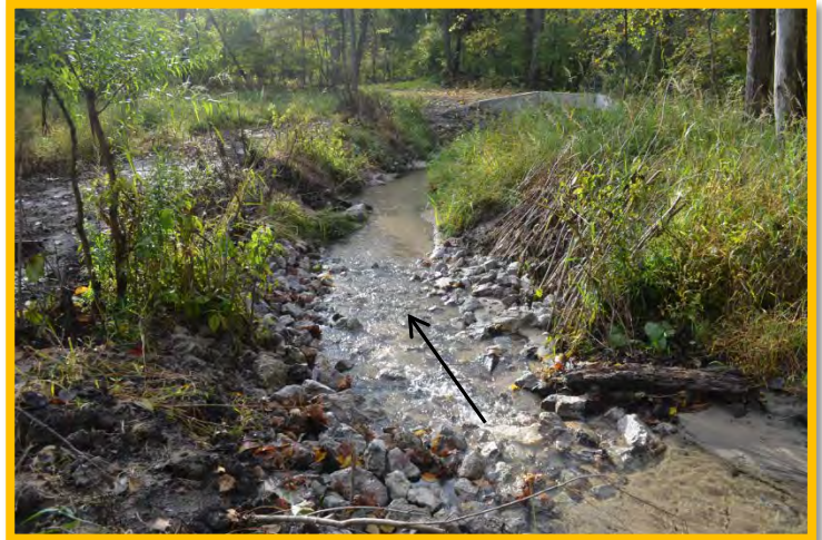
Image 2: Typical ERR. Designed to raise the bed of the stream up approximately one ft. Camp Miakonda in Sylvania, OH. Kyle Spicer
