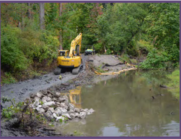
Construction begins by moving the stream bank material to position the LPSTP into a smoothed alignment.
