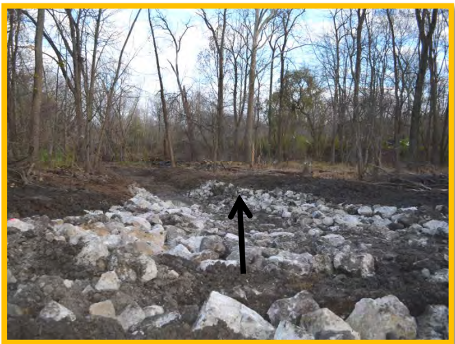
Finished ERR is sloped at 20 to 1, built of a well-graded, self-adjusting, self-filtering stone that was well-choked with smaller stone and gravel-cobble to fill in voids.
