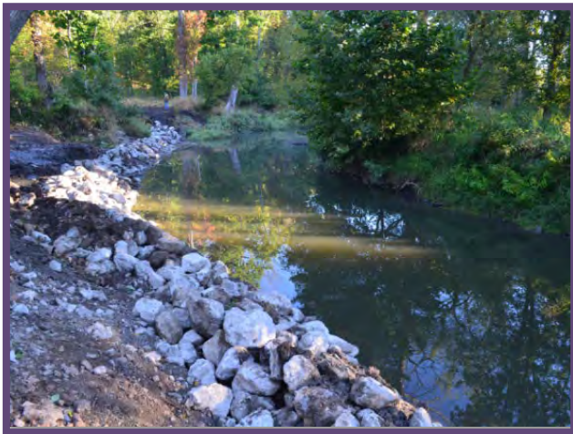
The area behind is then backfilled to create a contoured bank. The stone will self-adjust over times, further stabilizing the bank and looking more evenly contoured.
