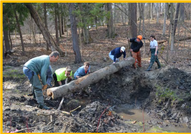
Image 3: Using a log to raise grade on Hartman Ditch. Rigid object (log was the only material on hand) was later undercut and failed, Camp Miakonda. Kristina Patterson.
