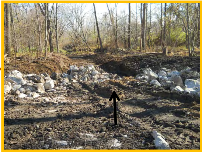
Bed protection of pool begins first, roughing in stone based on project needs (elevation control, fish passage [slope], and energy dissipation).
