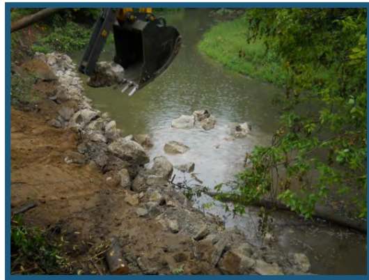
Construction begins by placing smaller stone as a filter, then buckets of well-graded stone. BW must be well-connected with the key stone.
