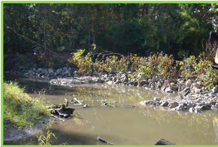
Image 1: Live Siltation installed over Longitudinal Peaked Stone Toe Protection at Camp Miakonda, Ottawa River. Kyle Spicer
