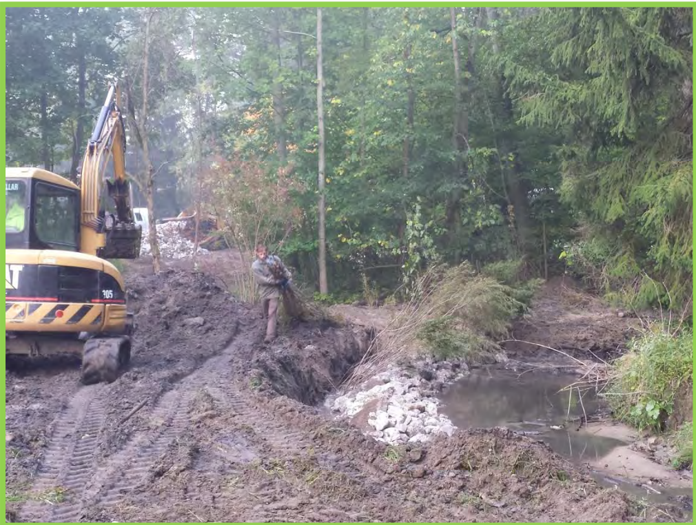
Image 2: Crews install Live Siltation at Camp Miakonda, Hartman Ditch, Sylvania, OH. Kyle Spicer.
