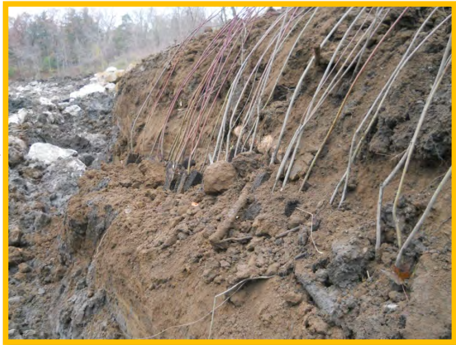
Bank protection starts with plugs and/or poles before it receives soil to cover base ends of poles, then stone will be placed.
