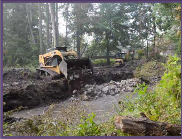
Stone is then deposited, depending on the size of the stream, over the bank with a skid loader or dump truck.
