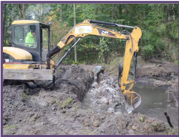
Excavator then positions the stone into the triangular shape, or otherwise if installing LFSTP. Behind the excavator’s work, Live Siltation is installed against the stone.
