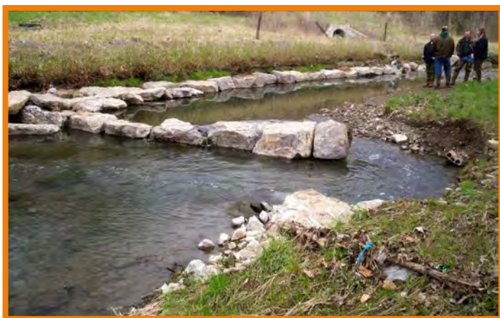
Image 1: A flanked grade control structure. Derrick
