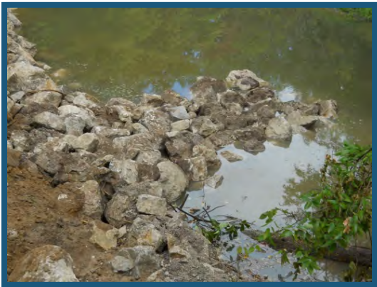
The typical BW has now taken shape. If fishing access is desired the BW can be top-choked with smaller stones and gravel.
