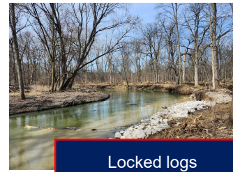
Bank Stabilization/ Re-grading
