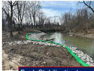
Bank Stabilization/ Re-grading
